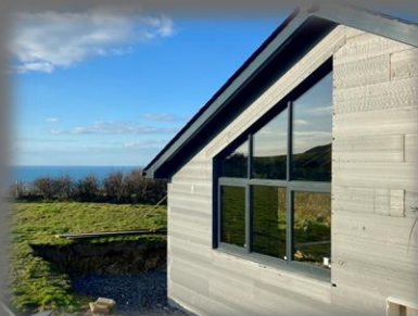
5. Install Roof, Electrics, Plumbing
