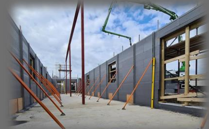
3. Add alignment brace system
