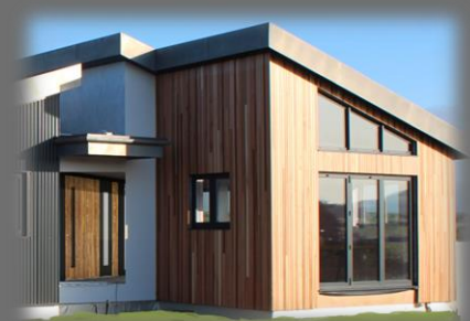
6. Apply Claddings, render and plasterboard
